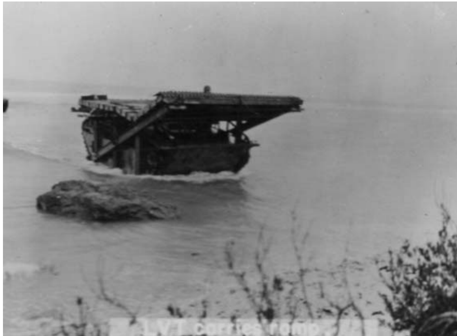
Figure 8.40. Doodlebug with ramp heading for the beach at Tinian, July 24, 1944. A portable ramp is attached to the top of this LVT. When it reaches the coral abutment, Seabees will jump out and attach the forward edge of the ramp to the coral cliff line. The amtrac then backs out, leaving the steel I-bars and the ramp behind. Tanks and other heavy equipment can then climb the ramp onto flat ground. US Navy, NARA.
