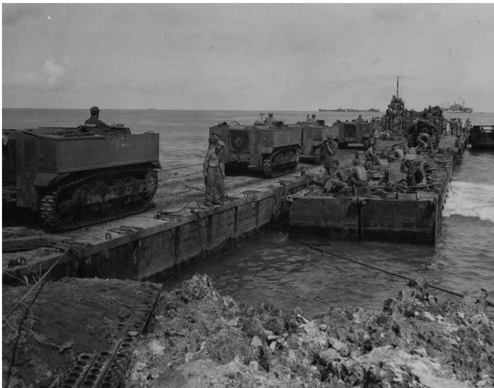
Figure 8.27. Pontoon barge and causeway at Chalan Kanoa erected by Seabees under fire. These pontoon causeways allowed LCTs to unload their tracked vehicles easily against rugged coral abutments. NARA.
