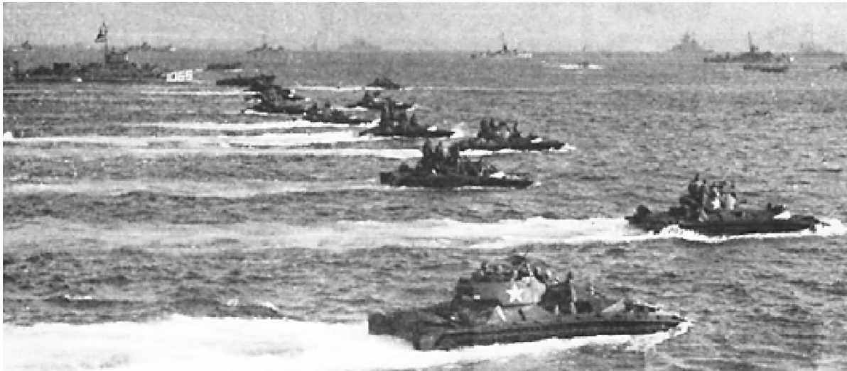
Figure 8.21. The armored Landing Vehicle Tracked (LVT) was over 26 ft long and could travel at speeds of 5.2 knots on the water and 25 mph on land. Various new models reached their full potential on Saipan, following their experimental use in the Marshall Islands. US Navy, NARA.
